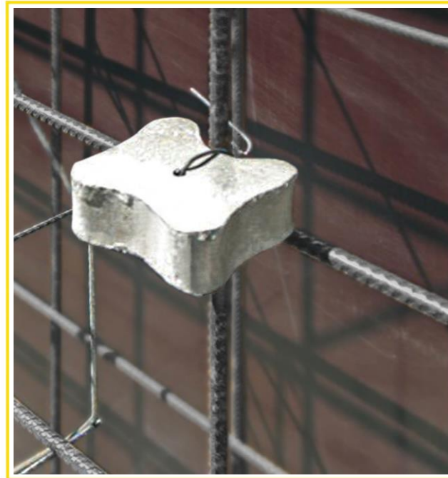
Glass Fiber Reinforced Concrete Spacers (GRC Spacer)
