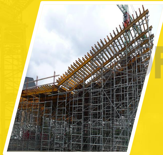
Concrete Slab Shoring Formwork (Staflex)
