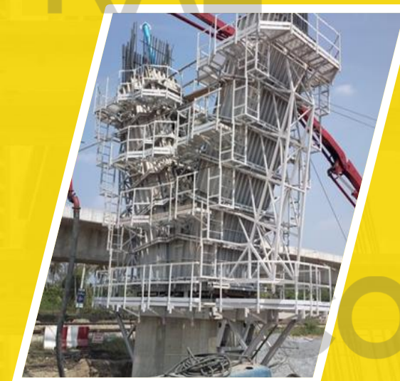
Formwork for Bridge Building
